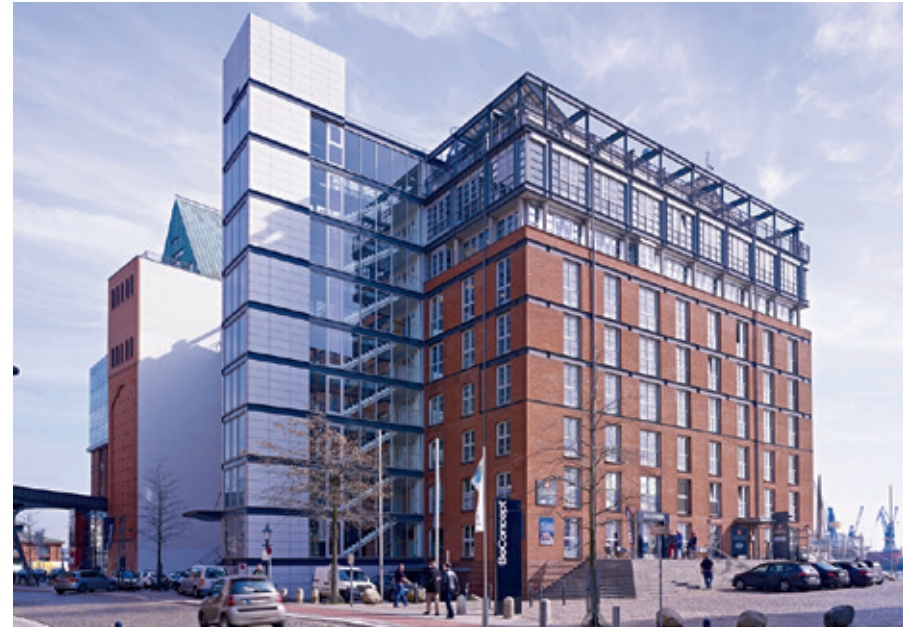
The GINN Hotel Hamburg will have more than 132 rooms over four former office levels when it opens in early summer 2017. This former warehouse located on the banks of the Elbe river also accommodates retail and office premises as well as a restaurant.
